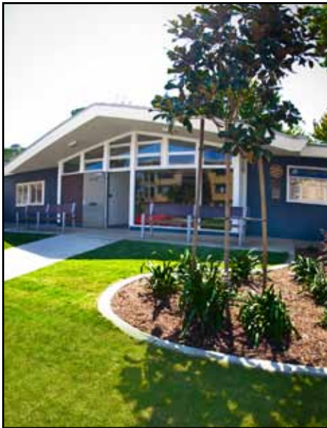
The Marine Street entrance to the school was transformed over the summer by BLOOM. Photo by Michael Spengler.
